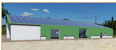
Centre Technique Municipal
